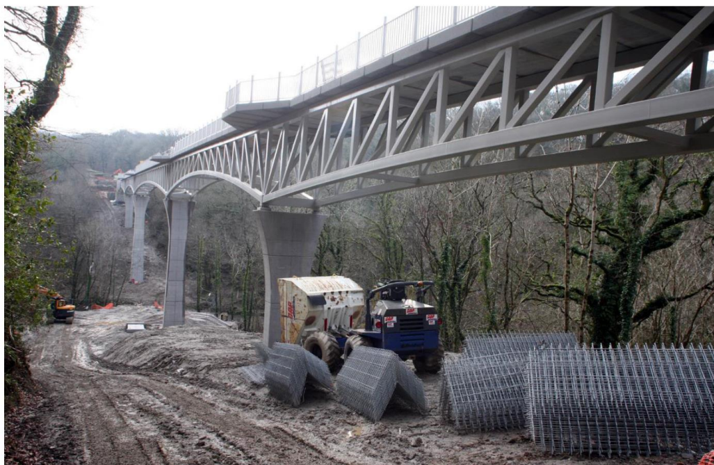
Gem Bridge (near Tavistock) Pedestrian / Cycleway 2013
