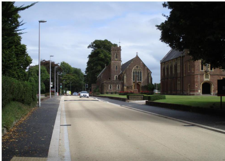
Completed Blundell's Road traffic calming improvements – October 2016
