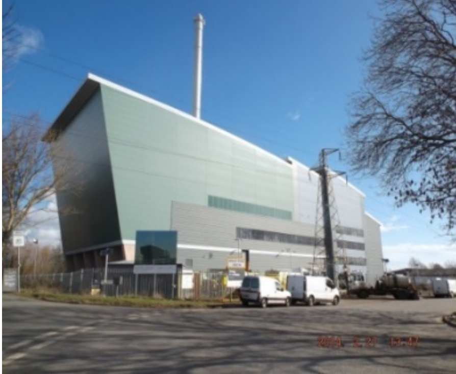
Exeter Energy Recovery Facility
