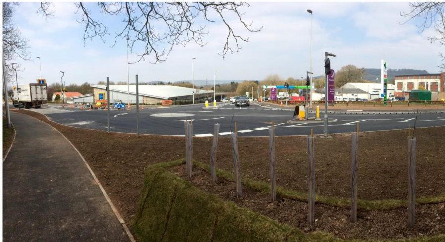
New mini-roundabout at Turks Head Junction in Honiton - March 2016
